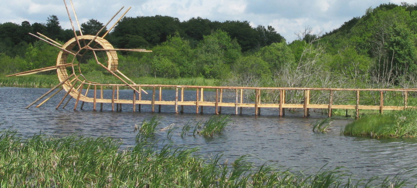
Back Flip Bridge (2009) - Wood (550 × 1850 × 80 cm); Massif du Sancy, France.
